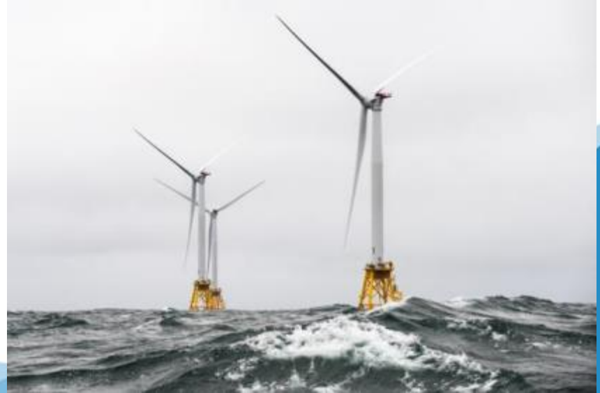
The Block Island Wind Farm—the first offshore wind farm in the United States. Photo by Dennis Schroeder, NREL 40389
