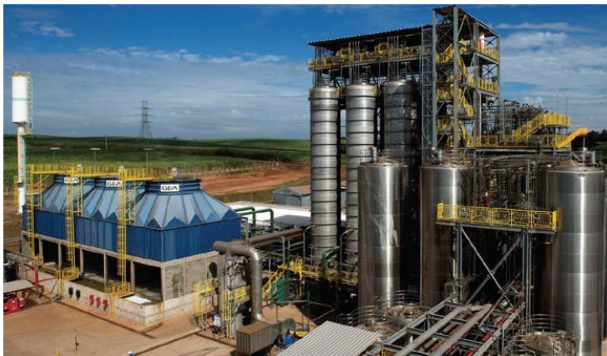
Figure 7: Amyris' facility in Brotas, Brazil uses bubble columns with external cooling loops (22). Source: Amyris, Inc.
