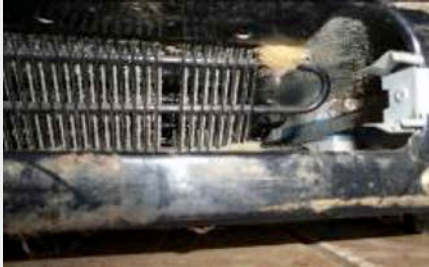
Vacuumed refrigerator coils (top: pre-retrofit; bottom: post-retrofit).
