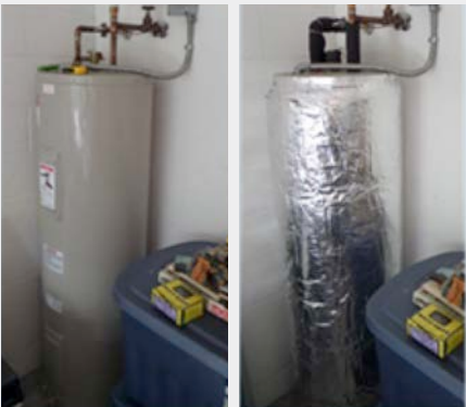
Hot water tanks and pipes were insulated (left: pre-retrofit; right: post-retrofit).
