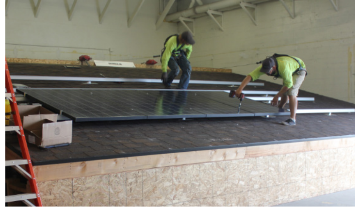
Figure 6. Second installation crew working on the Ironridge system
