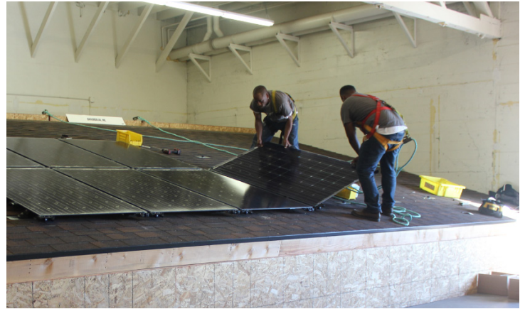
Figure 4. First installation crew working on the Ironridge system
