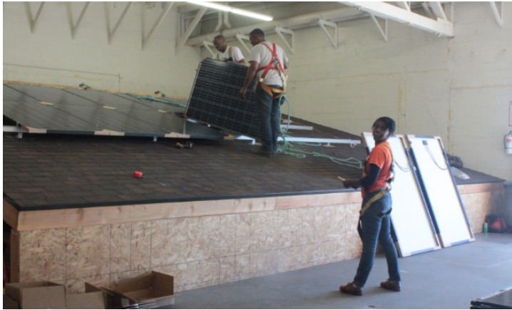
Figure 3. First installation crew working on the SMASHmount system
