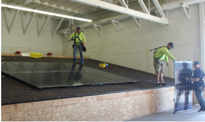
Figure 5. Second installation crew working on the SMASHmount system
