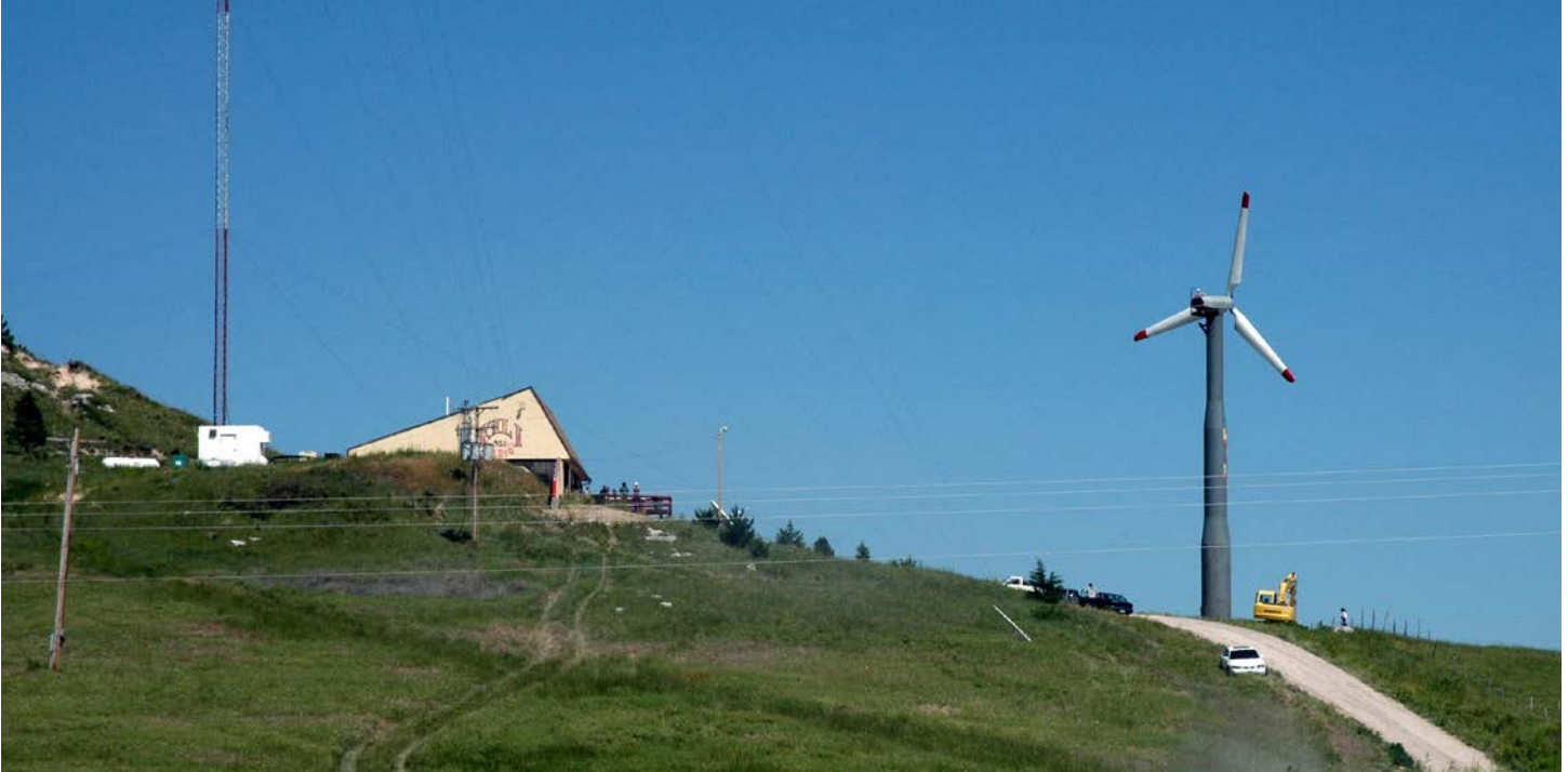
The U.S. Department of Energy's Office of Indian Energy provides financial assistance to federally recognized tribal governments and Alaska Native corporations to develop and deploy renewable energy projects on tribal lands. Shown here: a 65-kilowatt turbine supplies power to the Pine Ridge Reservation radio station in South Dakota. Photo by Bob Gough, NREL 16258
