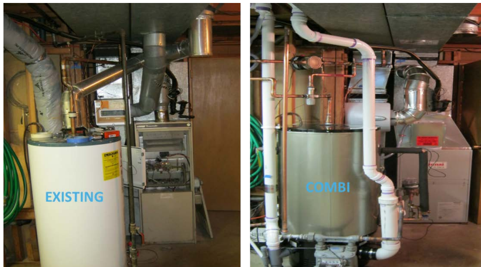
Figure 3. Comparison before and after installation
