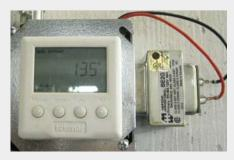
Supply temperature can be modulated with an aftermarket programmable control that is wired to the boiler and a temperature sensor mounted in a well in the DHW storage tank:
