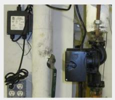
A demand control panel and recirculation pump are shown in the photo above. The control can accept either hard-wired pump connections or removable three-prong plugs. This flexibility simplifies the retrofit process.
