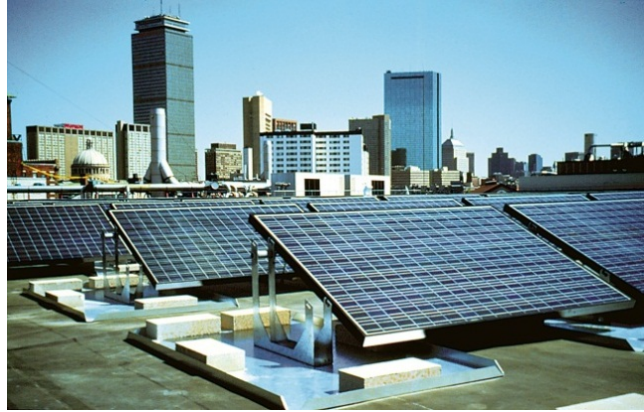
Source: NREL PIX 04478
