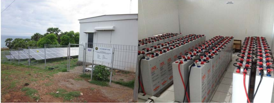
Figure 17. PV system with battery pack
