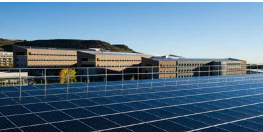
Image by Dennis Schroeder, NREL 27806
