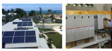
Figure 5. Left: Ocho Rios green community in Jamaica supports increased electric reliability through distributed solar and wind and microgrids. Right: A microgrid storage shed with batteries and inverters.
