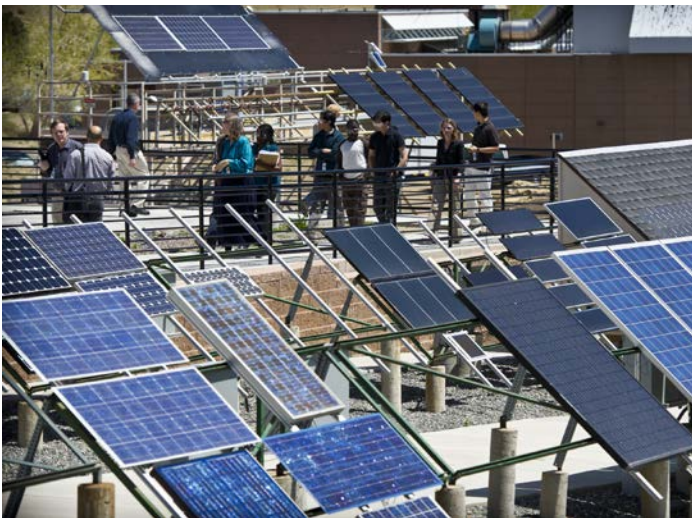
A variety of PV panels and systems are monitored under real-world conditions at NREL's Outdoor Test Facility. Photo by Dennis Schroeder, NREL 18921
