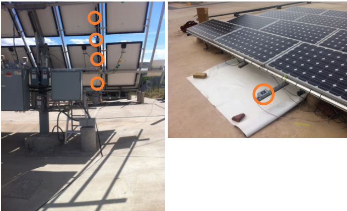
Fig. 2: Array 1 (left) is mounted 1 m above concrete at 40^\circ tilt. Array 2 (right) is a close-mount rooftop system at 10^\circ tilt above either beige or white roofing material. Front-facing irradiance is measured along with rearside irradiance at 3–4 positions (circles).
