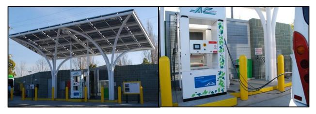
Figure 7. Bus fueling at the Emeryville hydrogen station: fueling area (left) and close-up of the bus dispenser (right)
