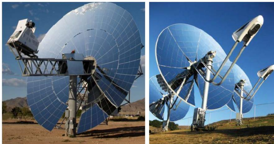
**Figure 12. Two types of dish/engine systems**
