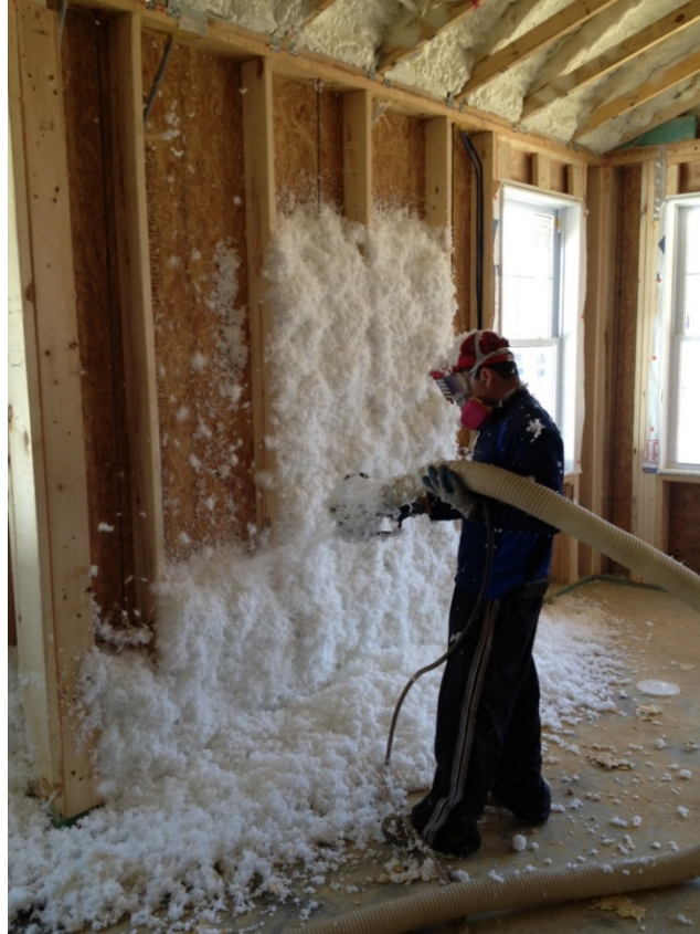
Figure 18. Installation of Johns Manville Spider insulation
