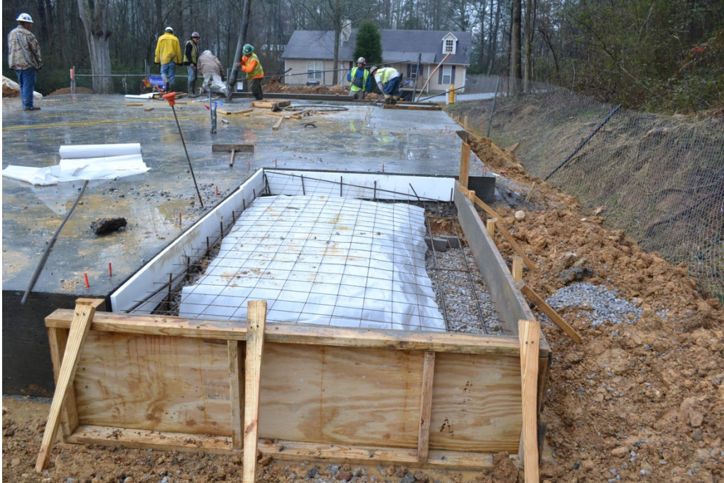
Figure 22. LaFayette slab edge insulation installed before the porch pour
