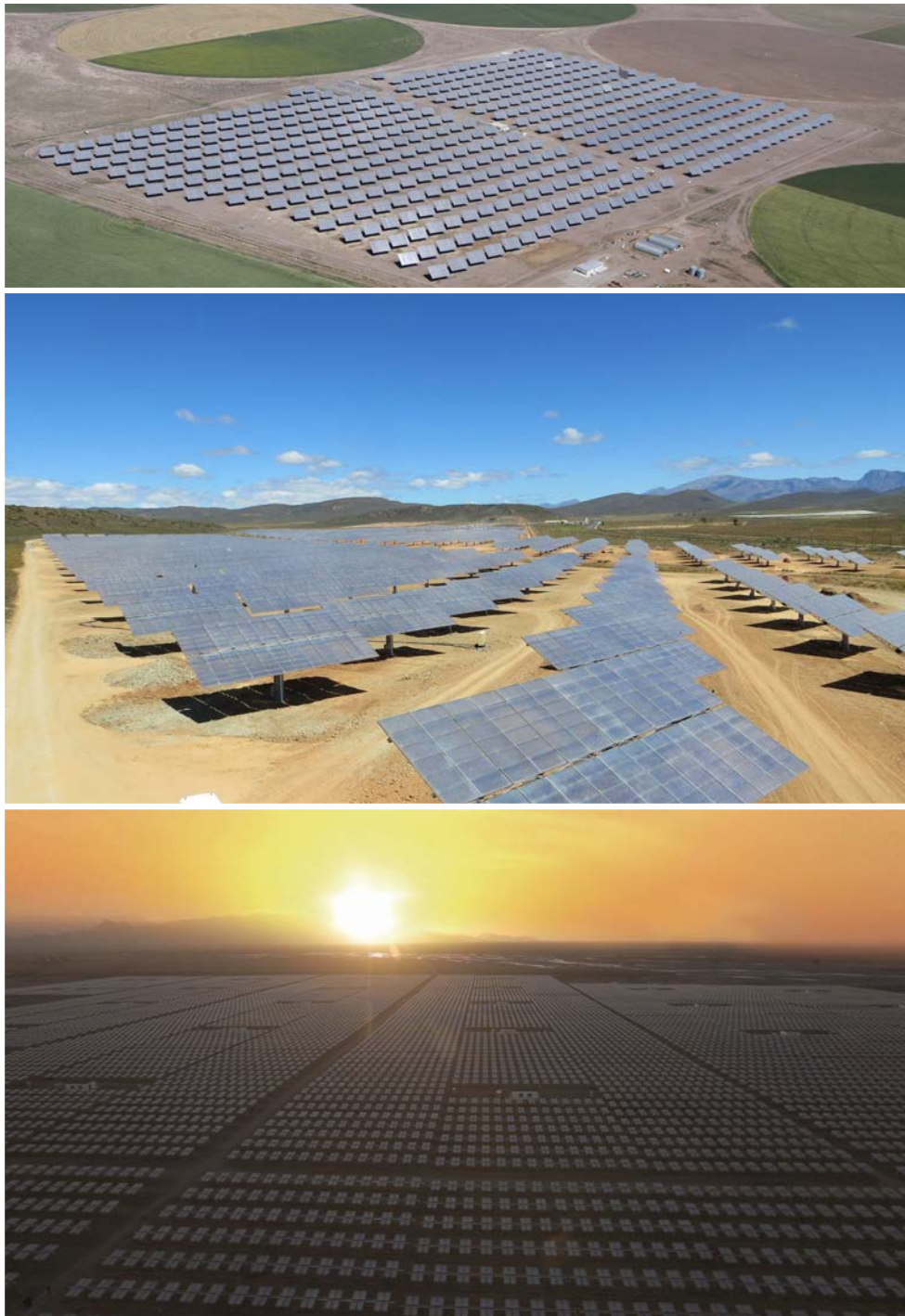
Figure 3: Examples of large CPV power plants. From top to bottom: 30 MW plant in Alamosa, Colorado, USA (© Amonix); 44 MW in Touwsrivier, South Africa (© Soitec); 140 MW in Golmud, China (© Suncore).
