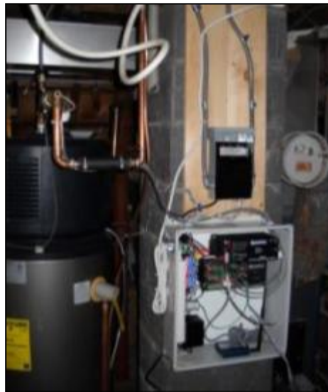
Figure 3. Example of an HPWH monitoring system installation
