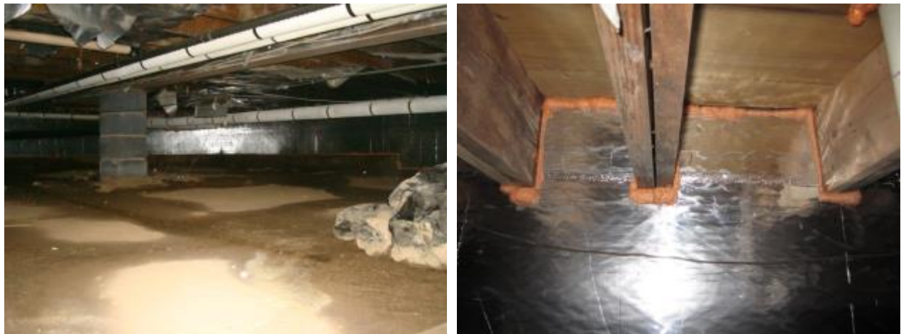
Figure 3. Postretrofit crawl space conditions (left); insulation board sealed at joist ends (right)
