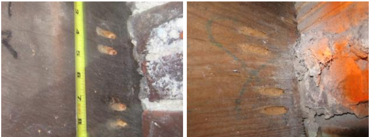
Figure 28. Wood color comparison at BSMT-E1 joist (left); FIRST-E joist (right)
