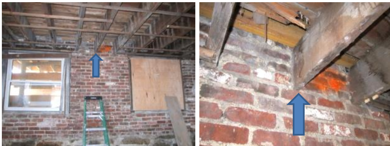
Figure 25. BSMT-E2 joist, showing existing water staining
