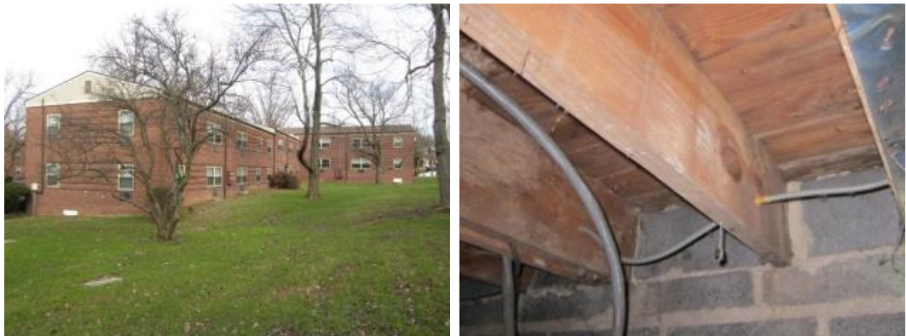
Figure 2. Overview of apartment complex (left); preretrofit joist ends in concrete masonry unit walls (right)
