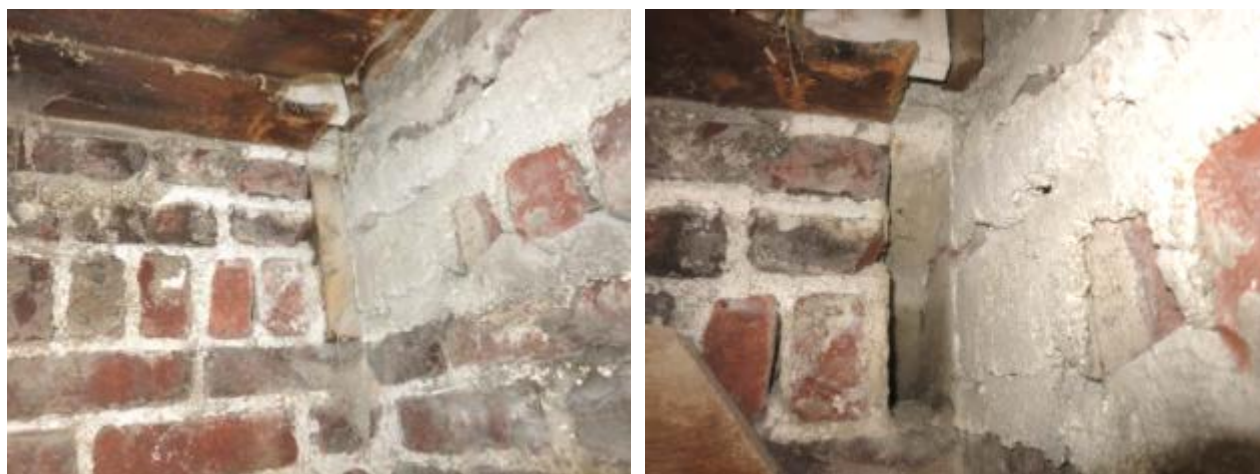
Figure 61. Joist end stub embedded in wall (left); joist pocket showing mortar (right)
