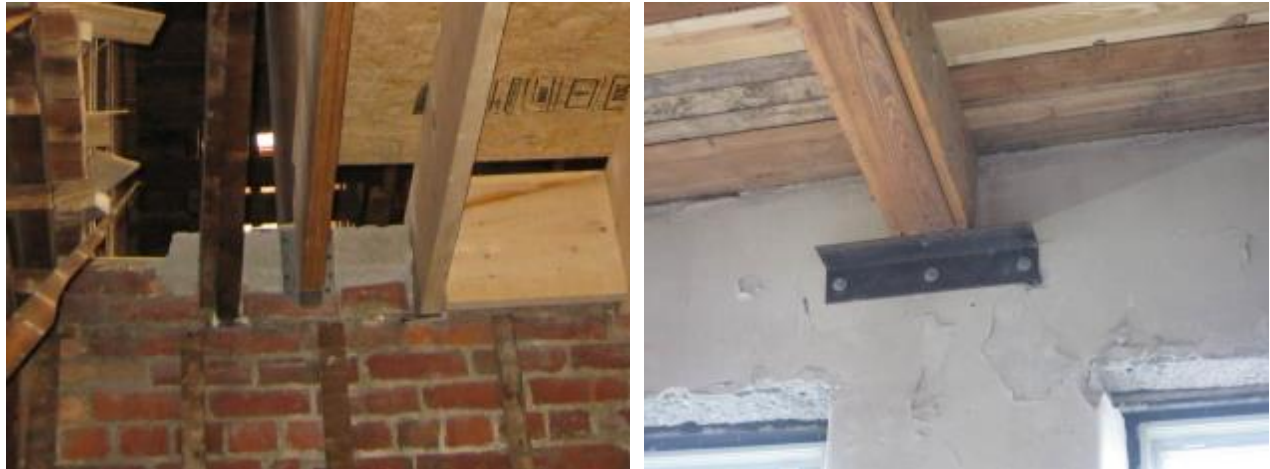
Figure 75. Transfer of load from masonry using joist hanger (left) or structural angle (right)
