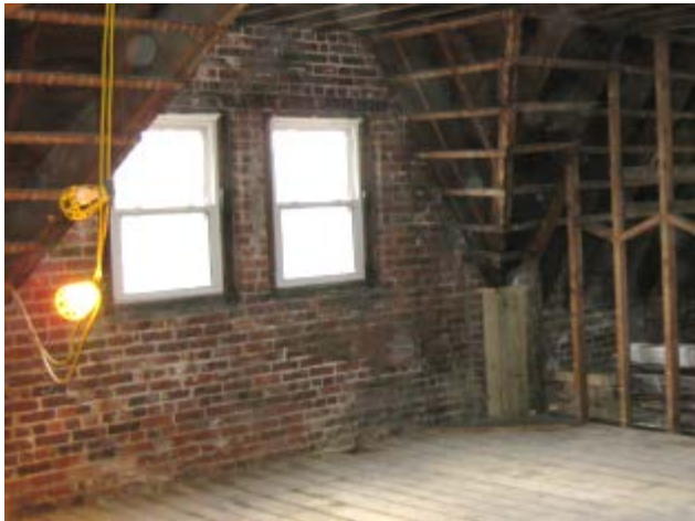
Figure 16. Exterior wall conditions at solid brick (left); hollow clay block infill (right)
