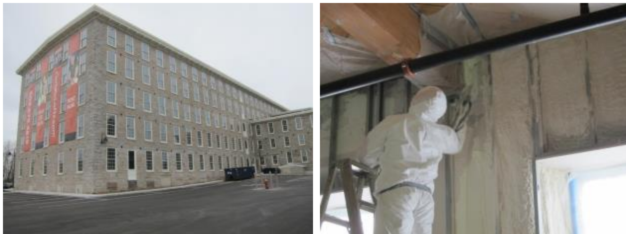
Figure 1. Mass masonry retrofit project overview (left); interior insulation at beam ends (right)
