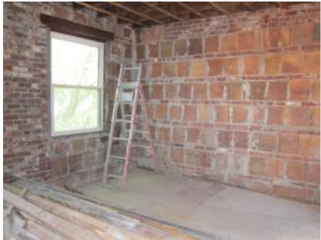
Figure 16. Exterior wall conditions at solid brick (left); hollow clay block infill (right)
