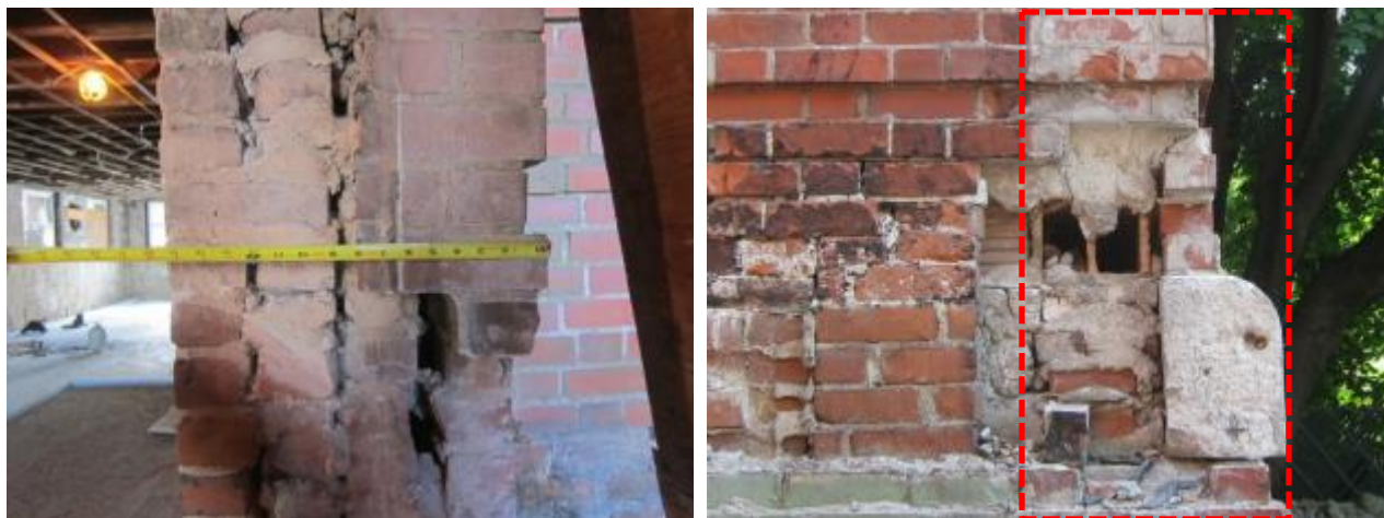
Figure 17. Wall section at solid brick (left); at hollow clay block infill (right) conditions
