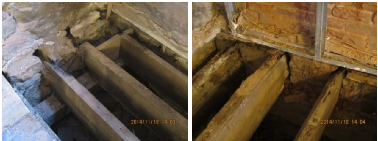
Figure 12. Damage to embedded beams at walls
