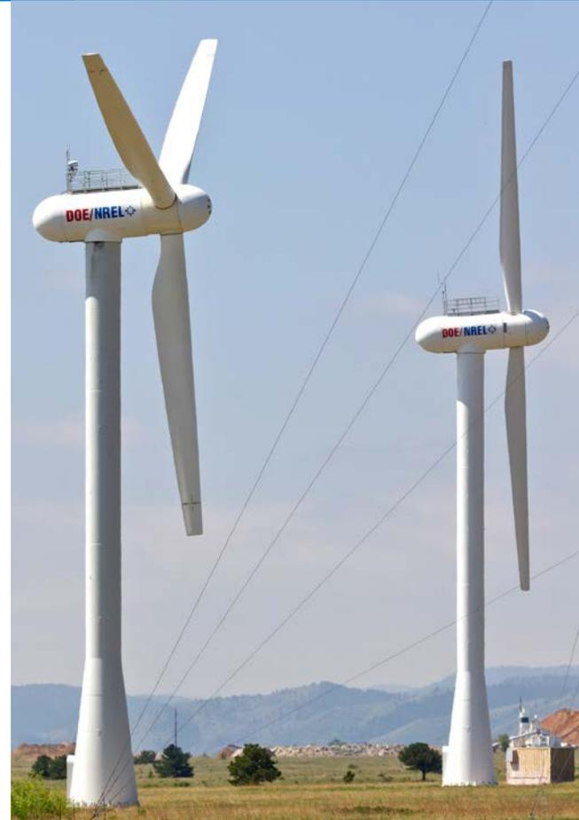
The NWTC's experimental wind turbines, a three-bladed Controls Advanced Research Turbine (CART3) and a two-bladed CART2. Both are used to validate new control schemes and equipment for reducing loads on wind turbine components.
