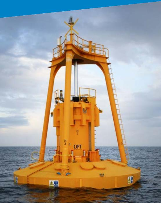
An example of a water power system that captures the energy of ocean waves, driving a generator to produce electricity. *Photo by Ocean Power Technologies, NREL 22857*
