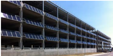
Fig. 4. NREL parking garage PV array
