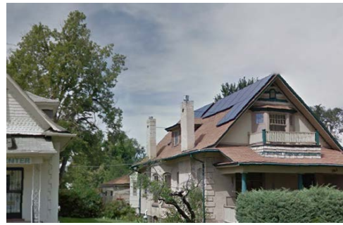
Fig. 6. Partially shaded PV array at a Denver residence. (Google Street View, 2014)
