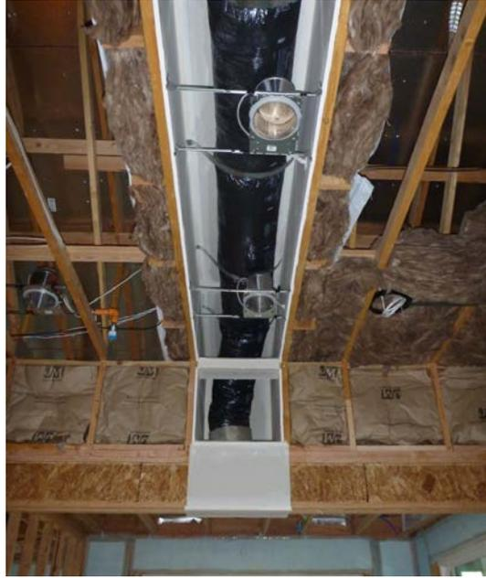
**Figure 4. Drywall-lined duct chase in the Wathan Castanos house**
