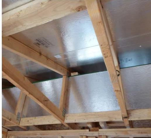
Figure 10. Exterior view of duct chase (1,816-ft<sup>2</sup> plan)
