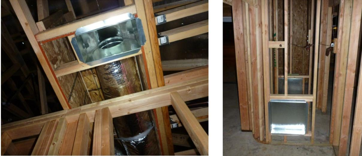
**Figure 13. Duct chase and boot for register (left); mechanical closet (right), Northwest Homes 2,205-ft<sup>2</sup> plan**
