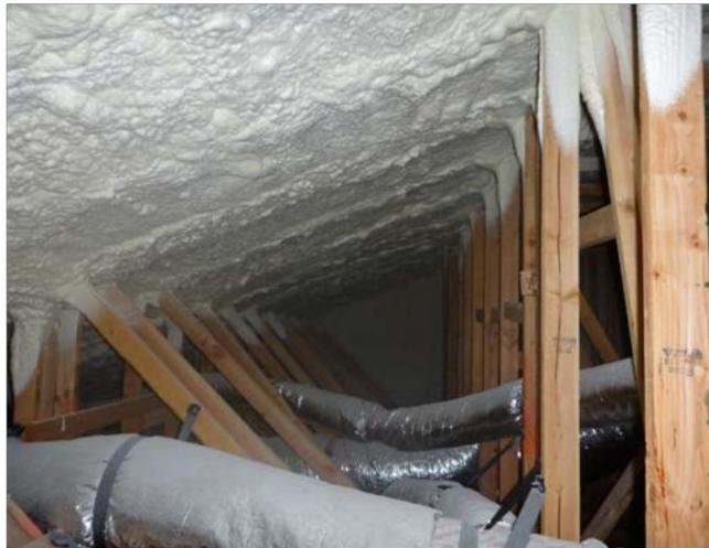
**Figure 3. Meritage's NVA with spray-foamed roof deck**
