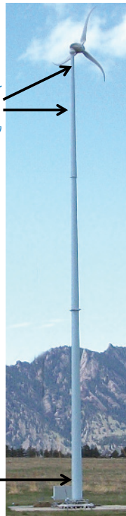
Figure 3. Test article used for full-scale loads measurement with identification of tower strain gage locations (Photo by Rick Damiani, NREL)
