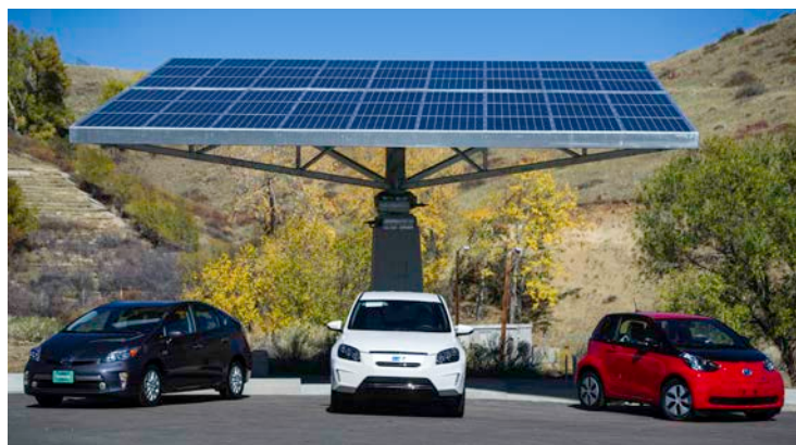
Electric vehicles parked under the solar tree charging system. Photo by Dennis Schroeder, NREL 22837
