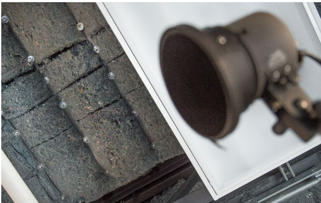
A recycled blue jeans product was purchased to insulate the photo studio on the STM campus as part of NREL's sustainability plan.
