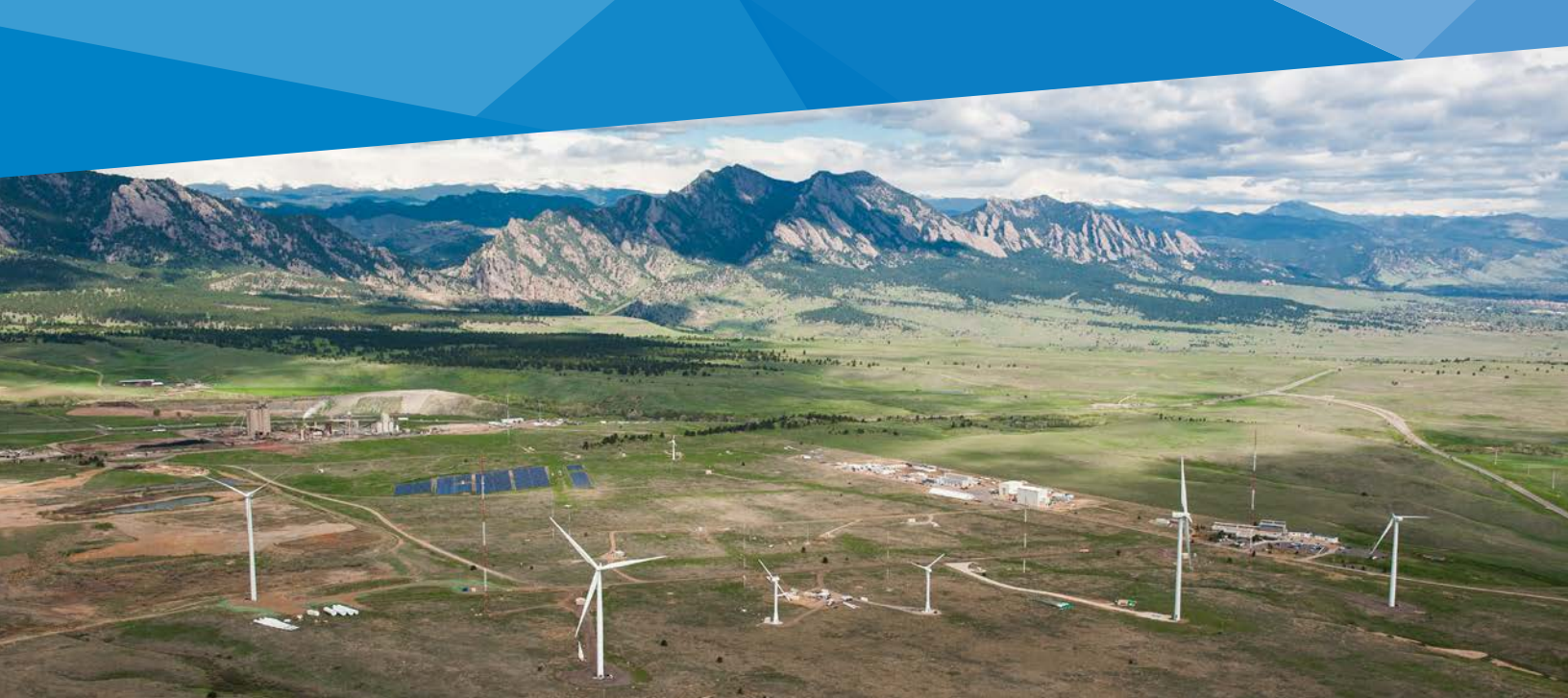
Aerial photo of the National Wind Technology Center (NWTC). Photo by Dennis Schroeder, NREL 25915
