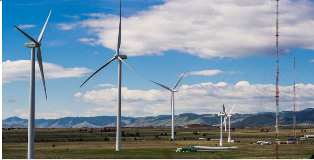
Aerial photo of the National Wind Technology Center (NWTC). Photo by Dennis Schroeder, NREL 25882
