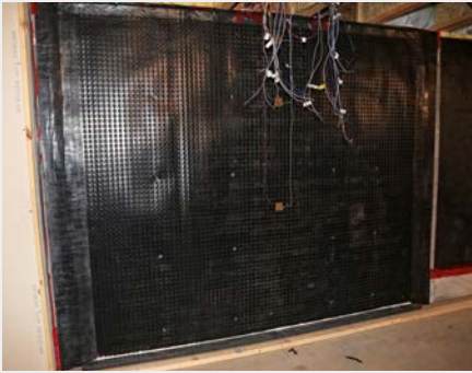
Nonadhered WSP with sealed perimeter
