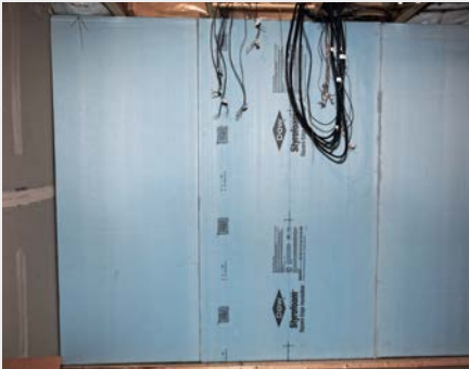
Rigid insulation with caulked joints
