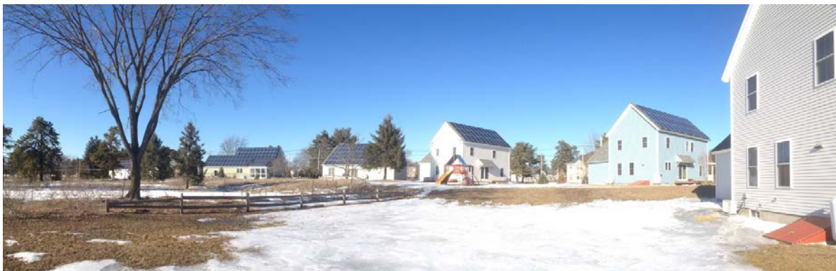
Figure 99. Overview of Devens site, showing PV arrays
