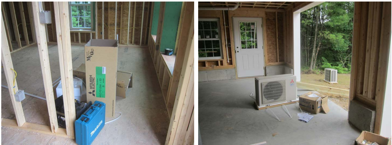
Figure 6. Unboxing and installation of MSHP equipment (Townsend, Massachusetts)
