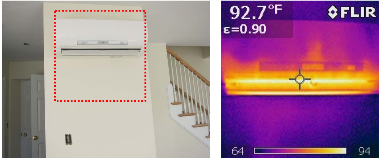
Figure 7. Indoor MSHP unit in heating mode, showing delivery temperature
