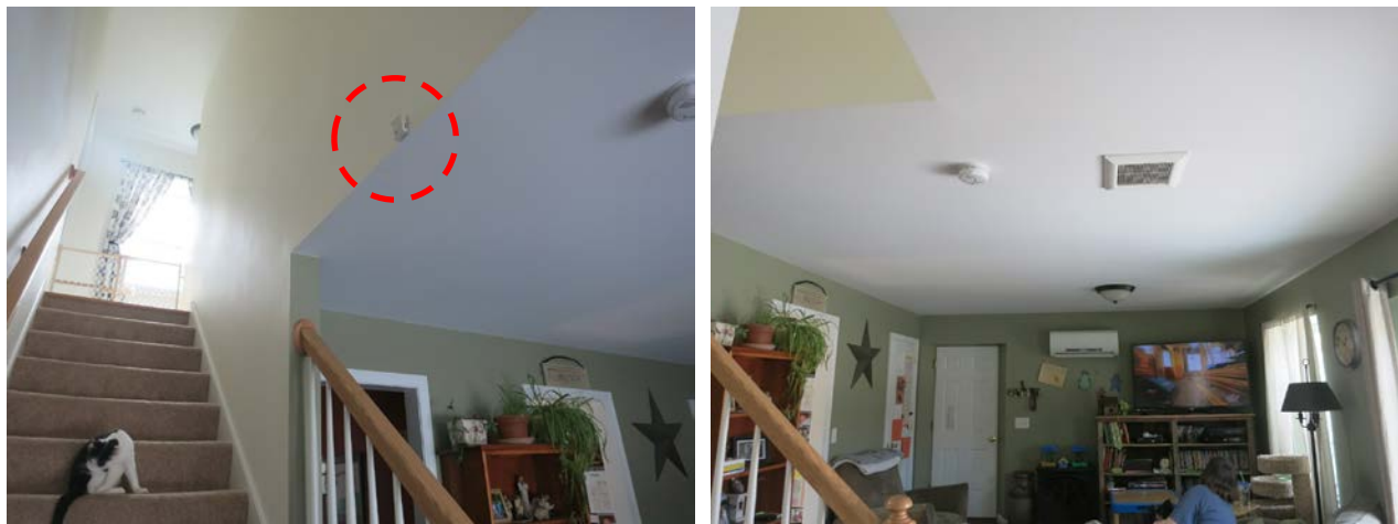
Figure 81. Easthampton Lot 17, view from base of stairs at first floor, stairwell temperature sensor highlighted
