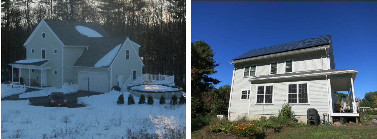
Figure 85. Easthampton Lot 30 front and south side views
