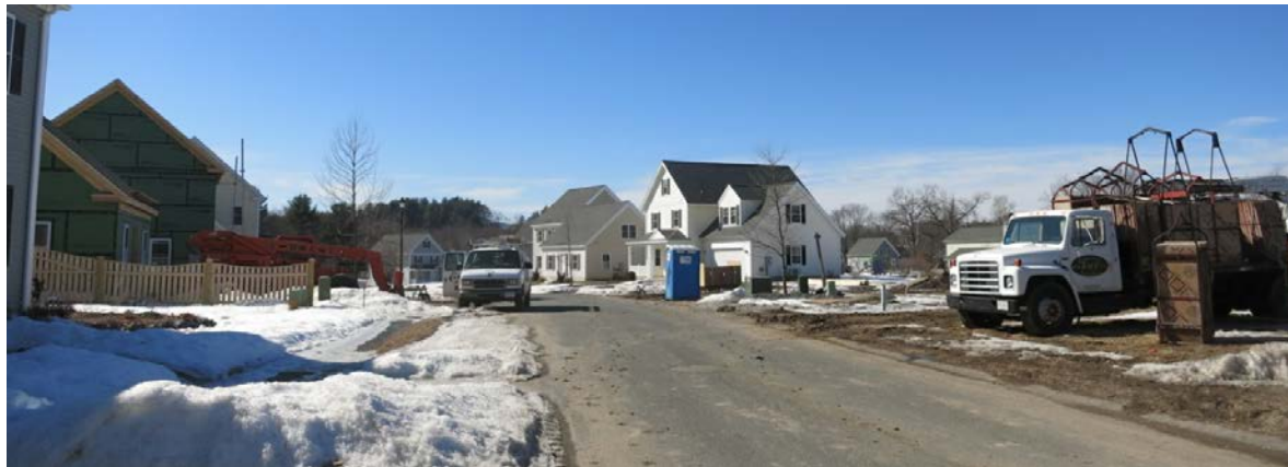
Figure 101. Overview of Easthampton site, showing continuing construction (March 2014)
