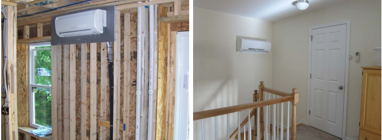
Figure 5. MSHP installation at house rough-in (L), and completed installation (R)
