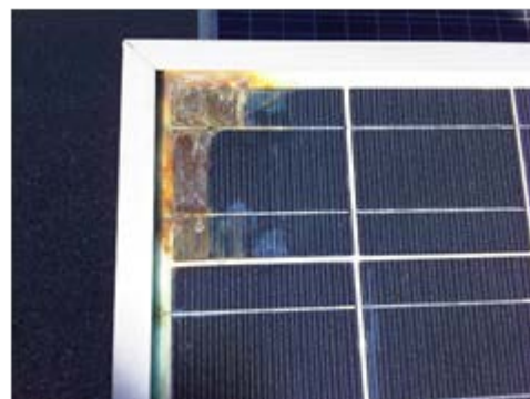
Figure 5: Corrosion of cell metallization from Arizona
