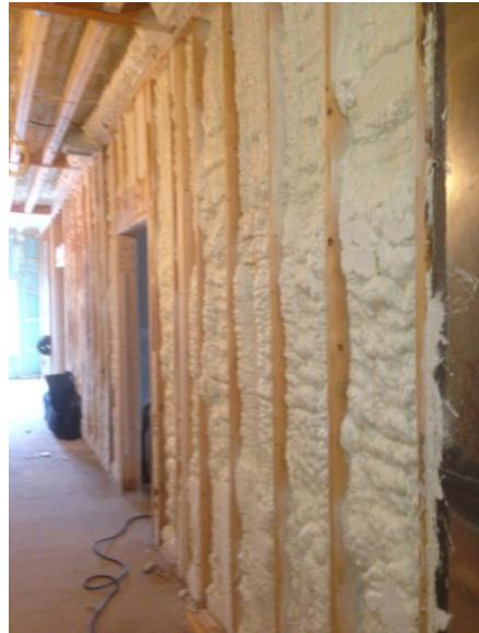
**Figure 11. Demising wall air sealing at HV**
