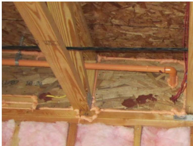
**Figure 8. Air sealed plywood smoke curtain used at demising wall of CV**
