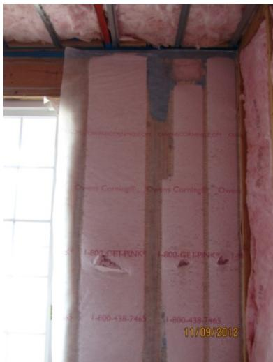
**Figure 6. Exterior wall air sealing and insulation used at CV and SH**
