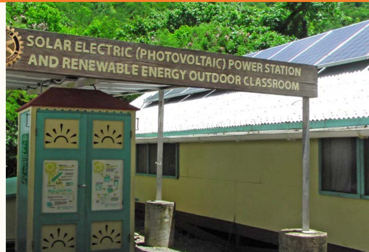
Almost 1,500 solar water heating and PV systems have popped up throughout the territory since the EDIN-USVI project launched in February 2010, and 15 MW of distributed solar PV are either in place or under construction. Photo from Don Buchanan, VIEO, NREL 20152
