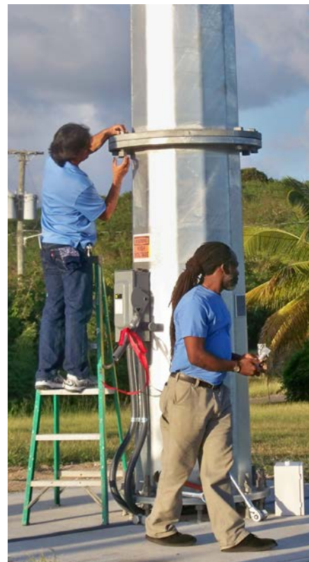
Workers install a 10-kilowatt wind turbine at the St. Croix Reformed Church and Kindshill School in St. Croix. Photo from Don Buchanan, VIEO, NREL 20418
