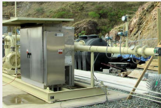
A landfill-gas-to-energy conversion system at Bovoni Landfill on St. Thomas will bring the USVI one step closer to meeting its clean energy goal. Photo from Don Buchanan, VIEO, NREL 20817
