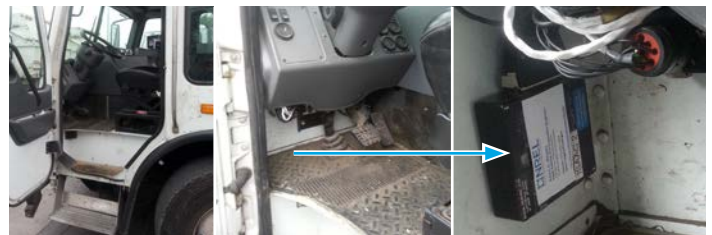
Data logger installation. Photos from Adam Ragatz, NREL 31125, 31126, and 31127
