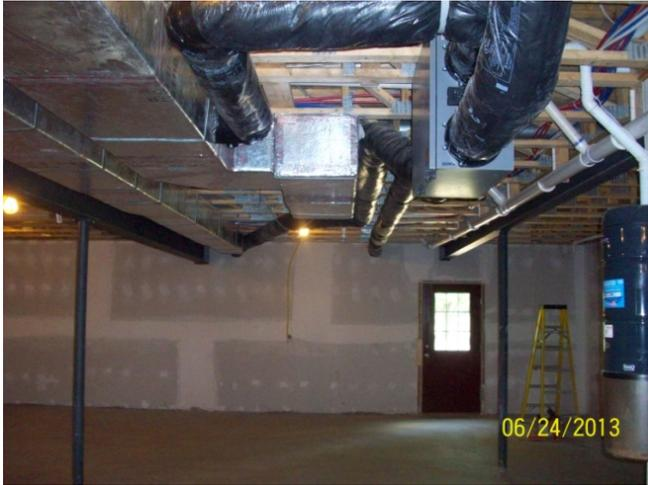
Figure 7. Duct system Installed in basement
