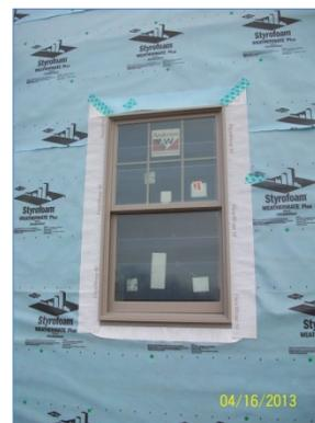
**Figure 17. Window flashing**
