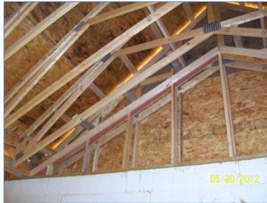
**Figure 22. Framed gable before air sealing and insulation**
