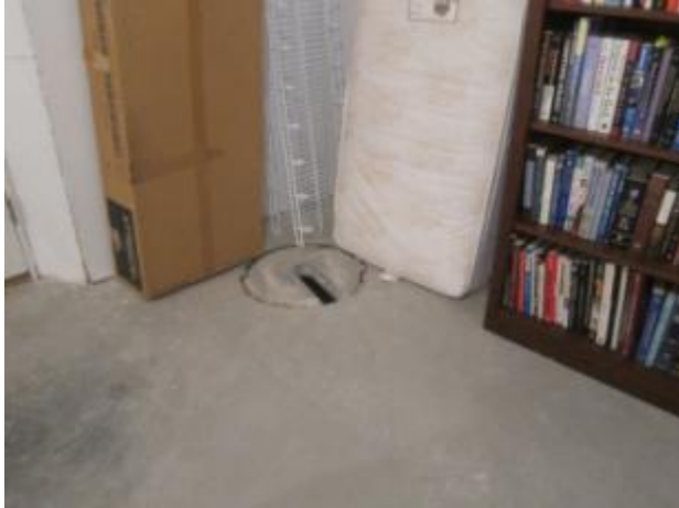
Figure 22. Plastic cover of sump pit, Lot 6
