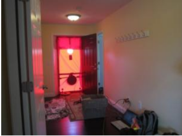
Figure 39. Depressurization testing of Lot 7
