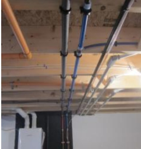
Figure 8. ¾-in. trunk at basement ceiling
