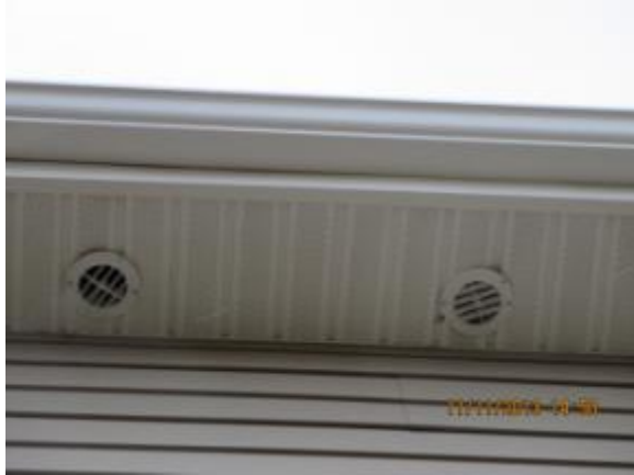
Figure 30. Second-floor bath exhaust terminations
