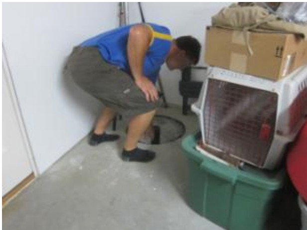
Figure 24. Plastic cover of sump pit, Lot 7
