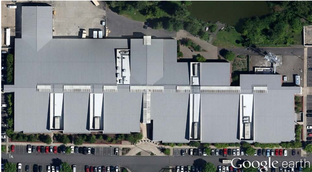
Figure 2. Aerial view of Anderson Readiness Center in Salem, Oregon
