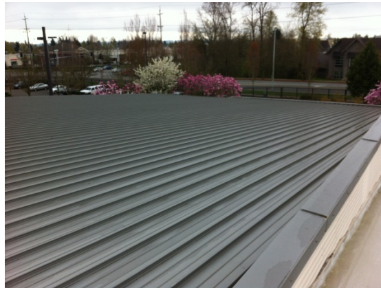
Figure 17. South-facing standing seam metal roof on the Salem ARC
