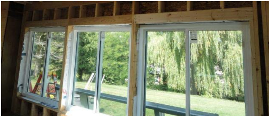
Figure 20. Window detail at built-out box
