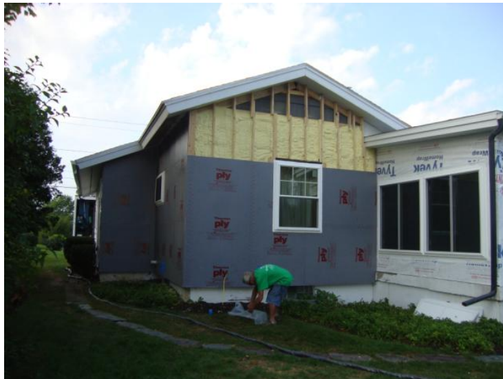
Figure 24. Exterior thin profile sheathing
