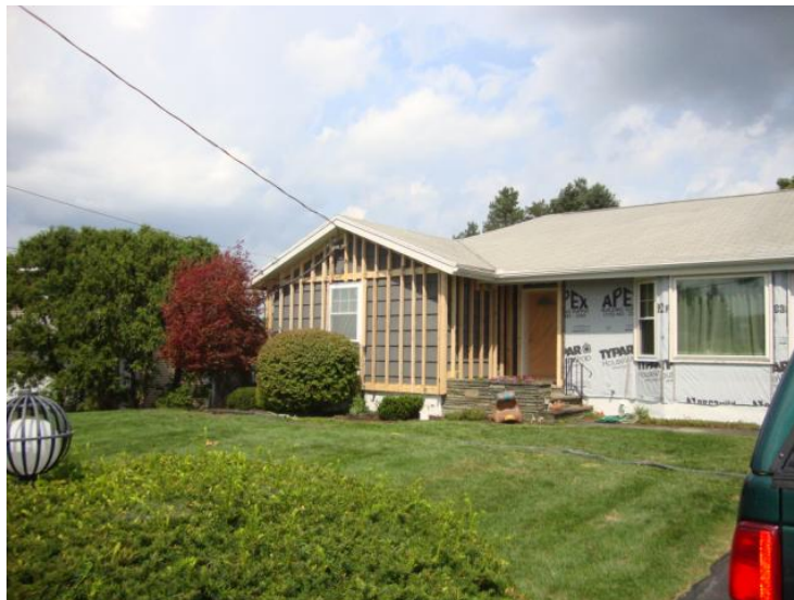
Figure 18. Exterior front framing
