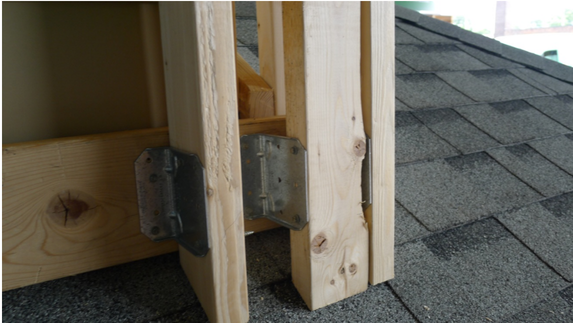
Figure 7. Simpson Strong-Tie “L” bracket
