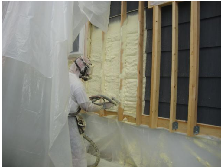
Figure 19. Installation of spray foam
