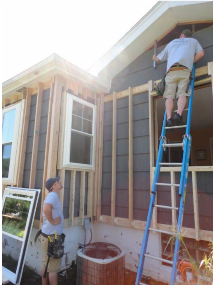
Figure 28. Installation of ledger boards
