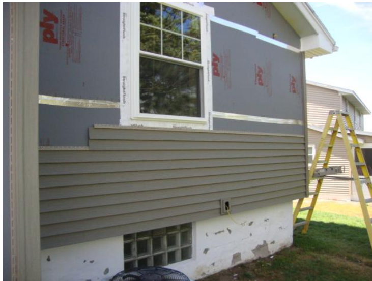
Figure 25. Siding Installation
