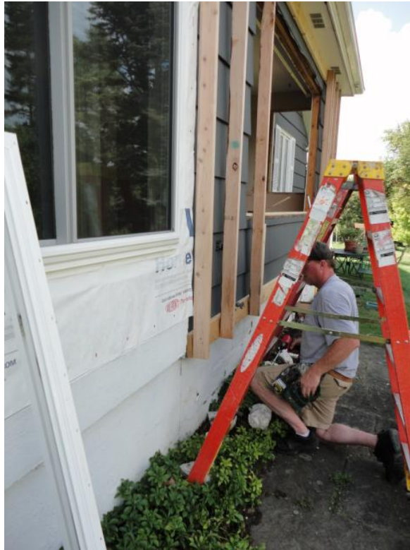
Figure 30. Window installation
