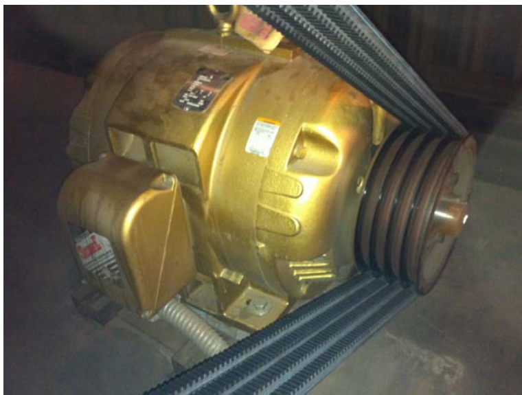
Figure 5 – VAV Fan Motor with Cogged Belts Installed. Image Credit: Jesse Dean (NREL)
