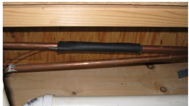
Figure 56. Typical surface mount thermocouple installation. Thermal paste, thermocouple, foam insulation tape, and cable ties if necessary.
