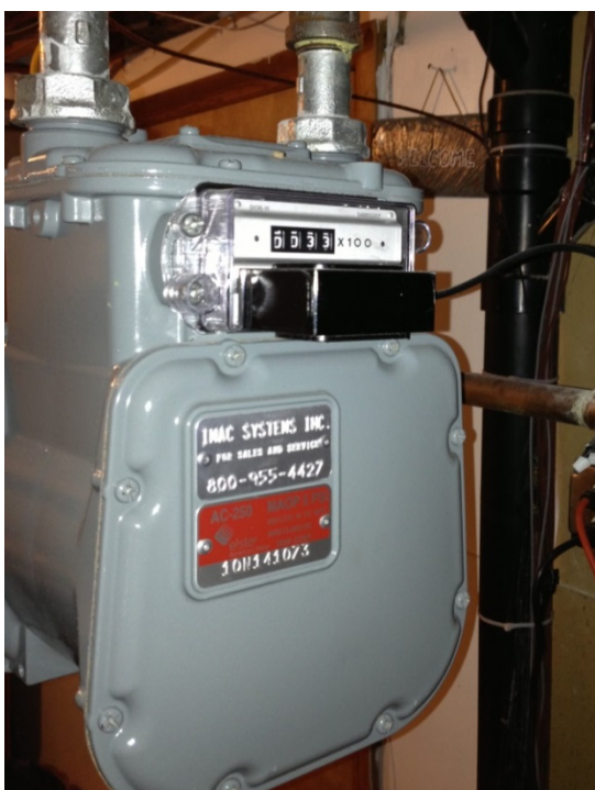
Figure 69. IMAC gas meter with pulser
