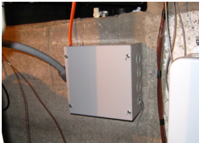
Figure 55. HPWH power is measured inside this enclosure. Inside are the CTs and power transducer.
