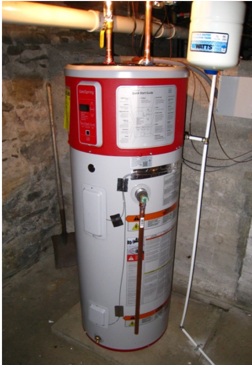
Figure 46. GeoSprings HPWH
