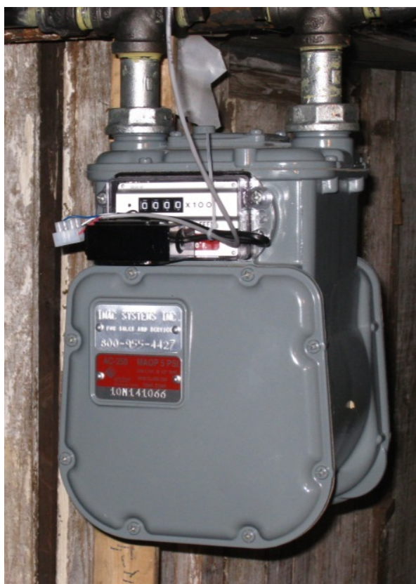
Figure 61. IMAC gas meter with pulser to measure gas use.
