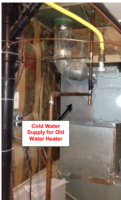
Figure 67. Original storage water heater location
