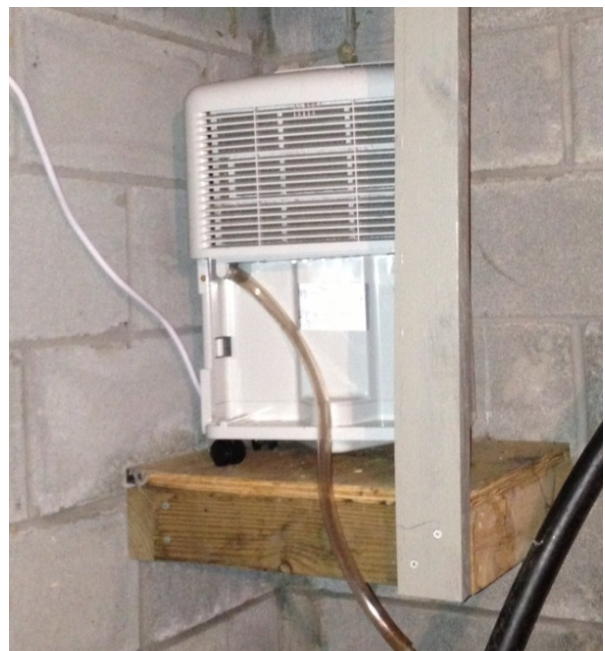
Figure 54. Dehumidifier in newer basement section with status and power being measured.
