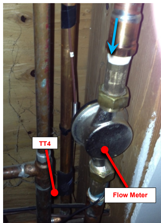
Figure 70. Flow meter and laundry trunk
