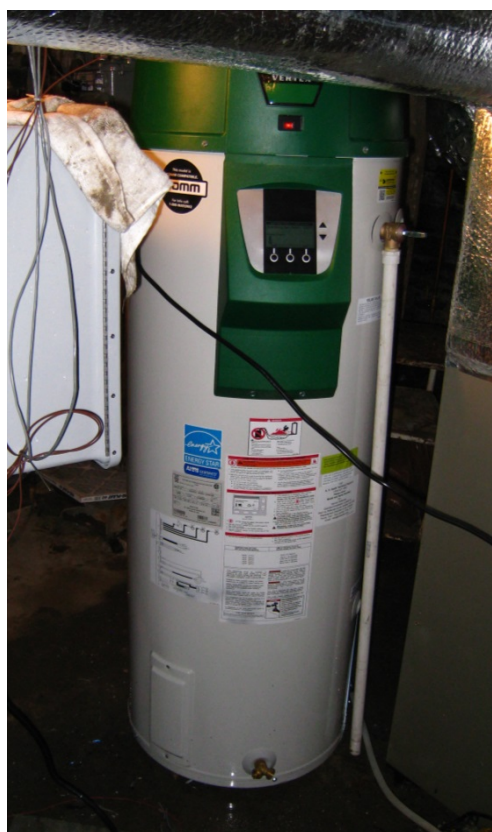
Figure 60. New condensing gas storage water heater installed during retrofit.
