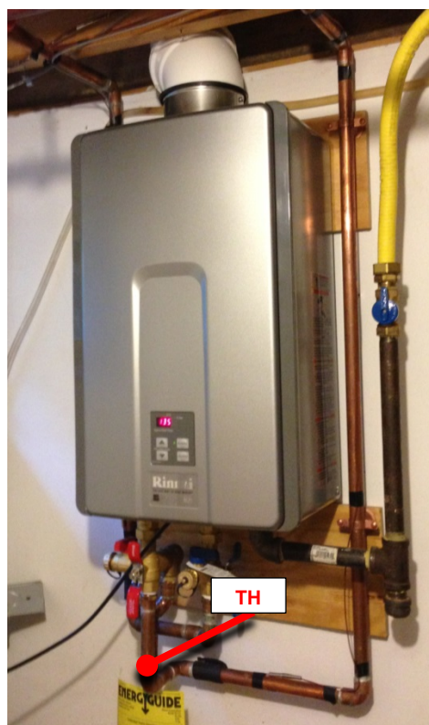
Figure 68. New tankless water heater from retrofit
