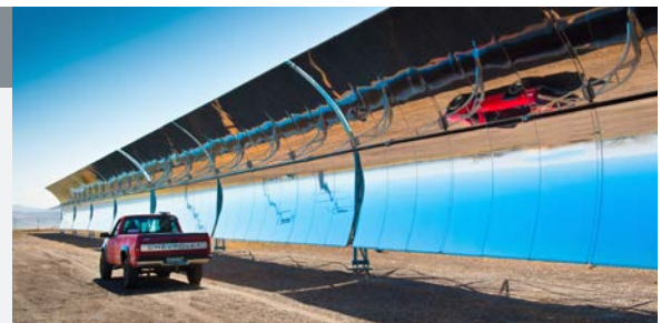
A pickup truck is equipped with Thermal Scout, which helps identify receivers in a parabolic trough plant that are losing heat and require maintenance. Photo by Dennis Schroeder, NREL 20336
