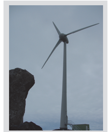
One of three Enercon E-33, 300-kW wind turbines installed as part of the Ross Island Wind Farm, providing power to the McMurdo and Scott Antarctic Research Stations as part of a medium contribution wind-diesel power system commissioned in 2010. Photo by Ian Baring-Gould, NREL 29393
