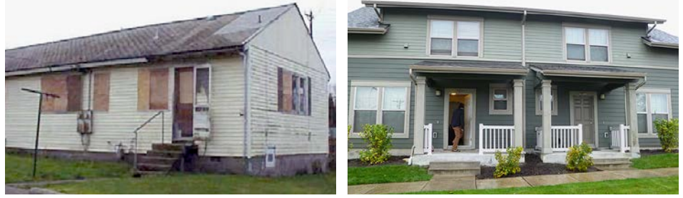
Left: Typical Salishan home prior to reconstruction. Right: New Phase 7 duplex in the Salishan development, built to ENERGY STAR standards by Walsh Construction.
