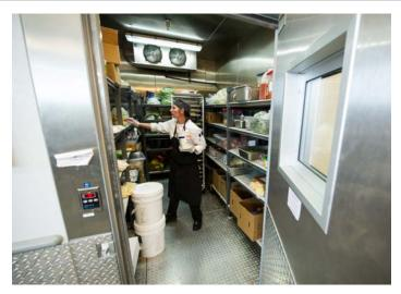
NREL's Café boasts energy efficiency features such as walk-in coolers and freezers that are equipped with door alarms, and LED lights connected to occupancy sensors that turn on and off automatically.
