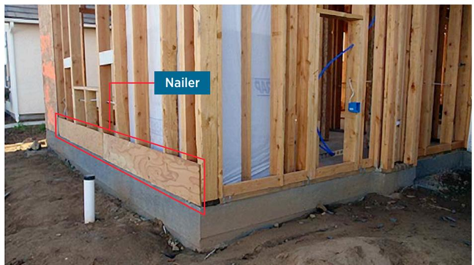
The slab edge of the test house prior to installation of the XPS rigid foam insulation, showing the nailer that supports the foam.
