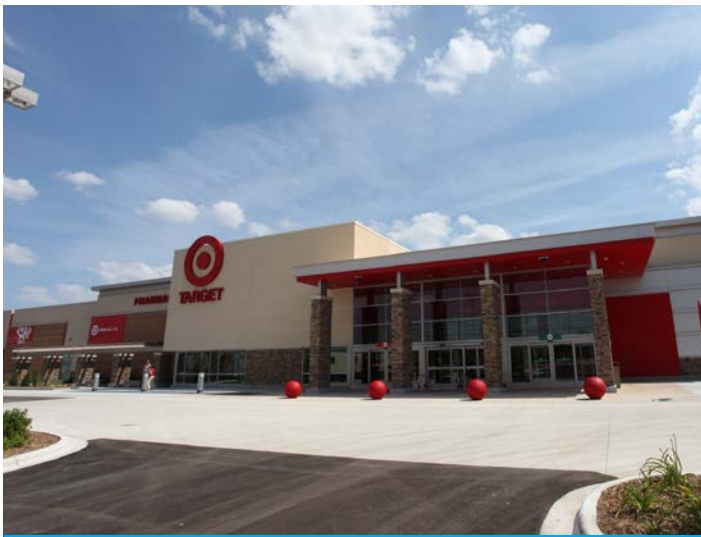
Image of the newly constructed Target store. Photo by Rois Langner, NREL 27648
