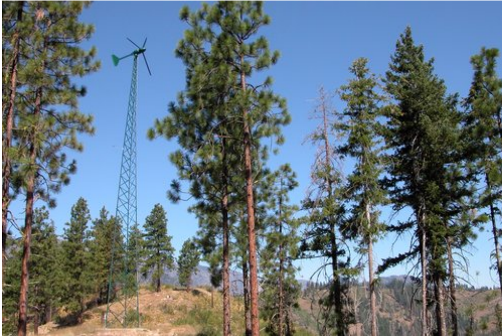
Poor site selection caused this residential Bergey 10-kW turbine to underperform significantly. Photo by Abigail Krich, NREL 13495
