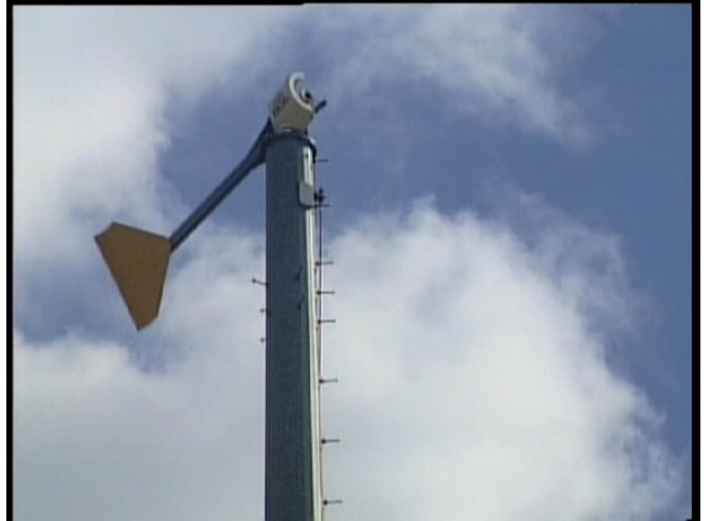
A Bergey 10-kW turbine at the Tom Ridge Environmental Center in Pennsylvania that was damaged in a storm. Photo by Lisa Adams, NREL 26432
