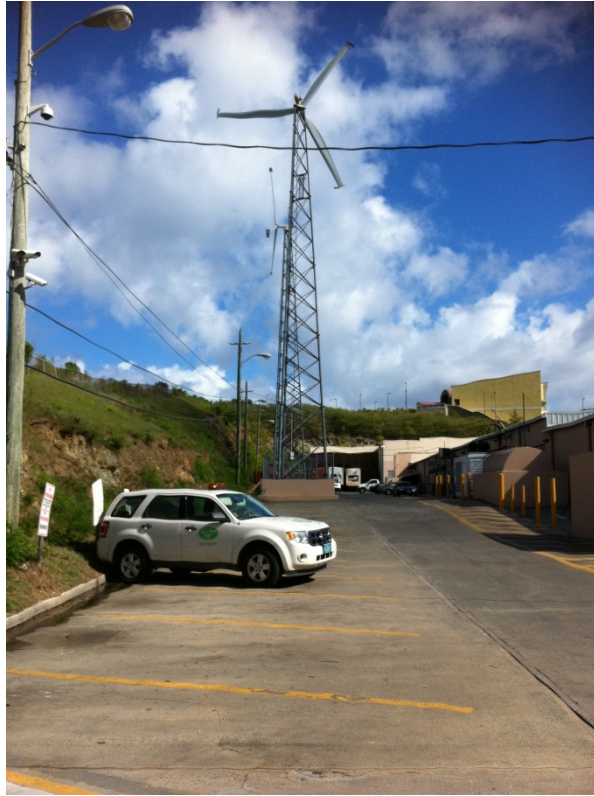
Poorly sited AOC 65-kW turbines in Tutu, St. Thomas, U.S. Virgin Islands. Photo by Owen Roberts, NREL 23839
