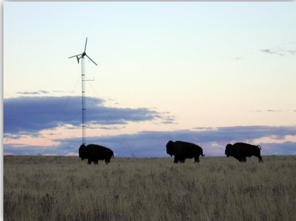
A Bergey 10-kilowatt (kW) wind turbine. Photo by Northwest Seed, NREL 13162
