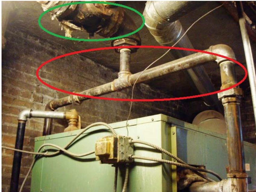
**Figure 4. The header piping is smaller than the boiler manufacturer’s specifications.**
