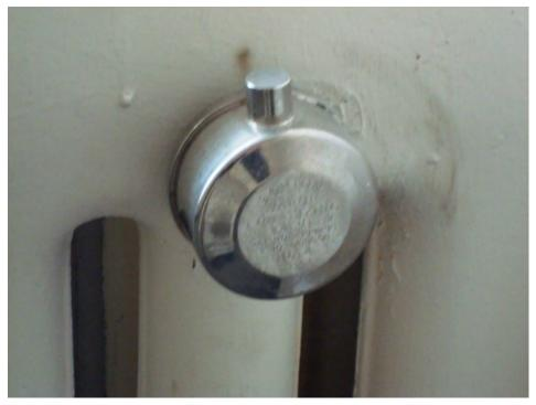
Figure 6. Gorton No. 4 angle radiator vent. Gorton models are made in No. 4, 5, 6, C, and D, ranging from 4 with the smallest orifice to D with the largest.
