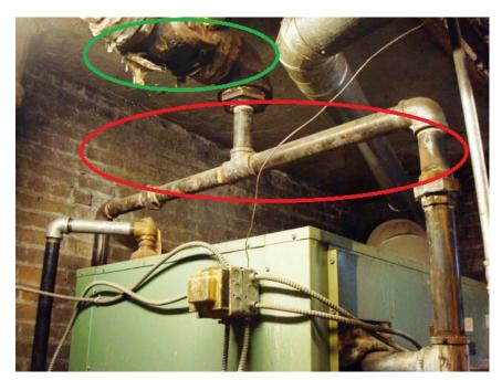
$\label{lem:figure 4.} \textbf{ The header piping is smaller than the boiler manufacturer's specifications.}$
