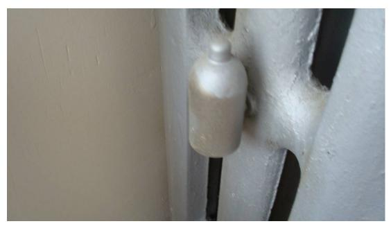
Figure 7. Painting over radiator vents is a common oversight that can have a serious effect on the heating in an apartment. Blocked radiator vents must be cleaned or replaced.
