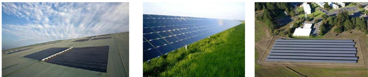
**Figure 4. Thin-film solar panels installed on (left) solar energy cover and (middle and right) fixed-tilt mounting system. Pictures from (left) Republic Services, Inc., 23817; (middle) Beck Energy, NREL 14726; and (right) U.S. Coast Guard Petaluma site, NREL 17395**
