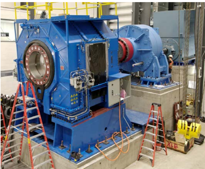
New dynamometer test facility under construction at the NWTC. Photo by Mark McDade, NREL 24472
