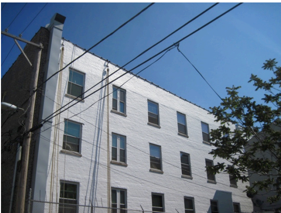
Figure 13. (L) Elastomeric paint application at larger multifamily building. Note that sills of windows are not painted; (R) Elastomeric paint application at two family building. (Credit: Scott Sanders, CEDA)
