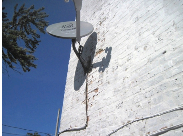
Figure 15. (L) Water and air control layer discontinuous at location of removed electrical conduit (blue circle) and gutter brackets; (R) satellite reception dish and associated cables create areas that will require touch-up to establish a continuous control layer with the elastomeric paint (Credit: Scott Sanders, CEDA)
