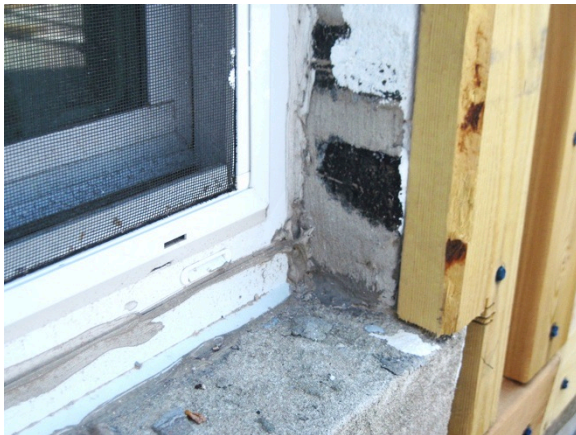
Figure 16. (L) Window in masonry opening with previously applied sealant; (R) new sealant and elastomeric paint applied at window opening. Note persistent gaps at transitions. (Credit: Scott Sanders, CEDA)
