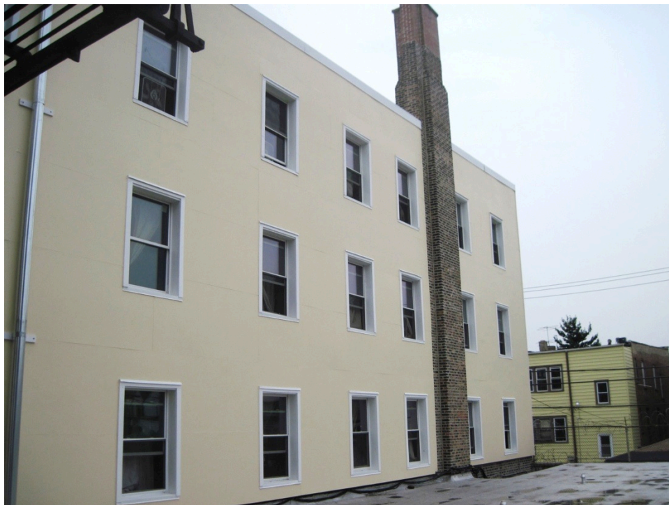
Figure 48. Finished side of the larger building
