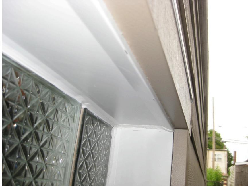
Figure 47. Window head return trim with profile channeling water to weep holes at the front edge
