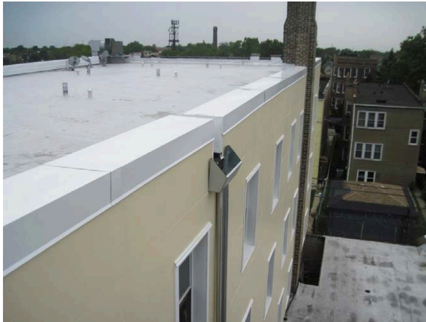
Figure 53. Visible butt joints in the finished wall
