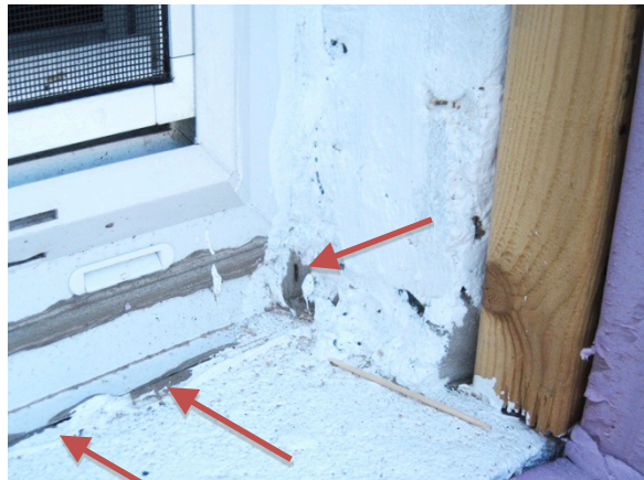
Figure 16. (L) Window in masonry opening with previously applied sealant; (R) new sealant and elastomeric paint applied at window opening. Note persistent gaps at transitions. (Credit: Scott Sanders, CEDA)
