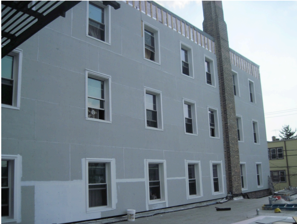
Figure 51. Caulked butt joints between 4 × 8 panels
