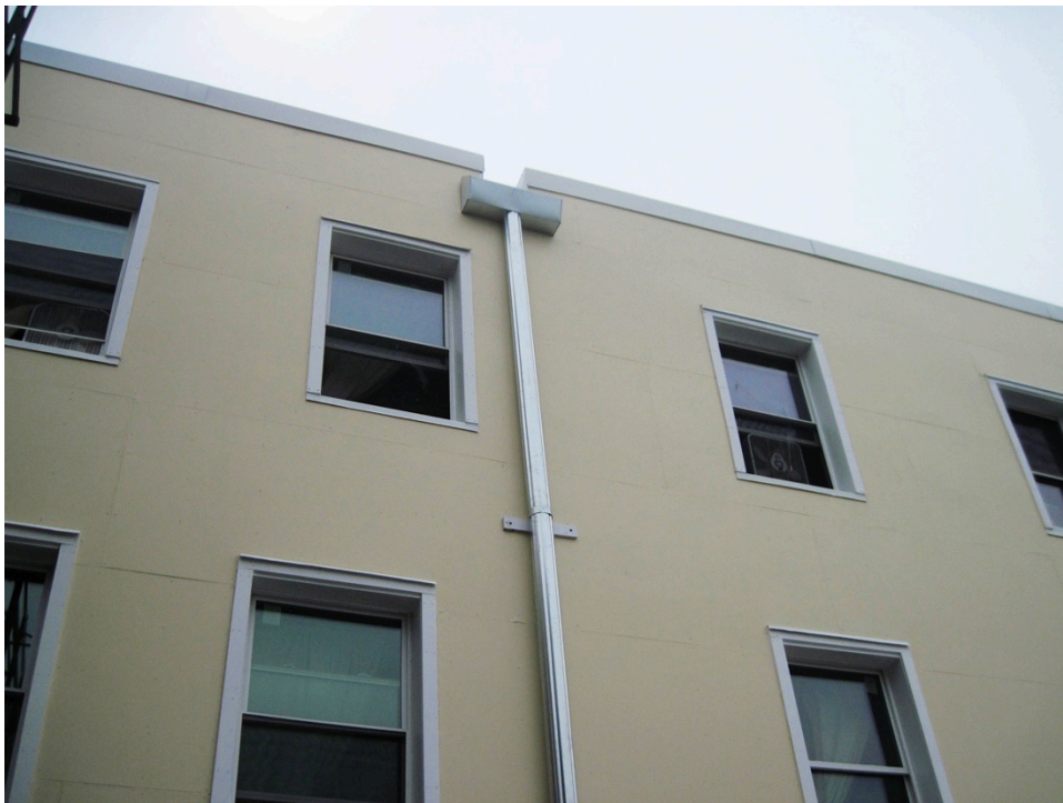
Figure 52. Butt joints between the panels visible in the finished wall
