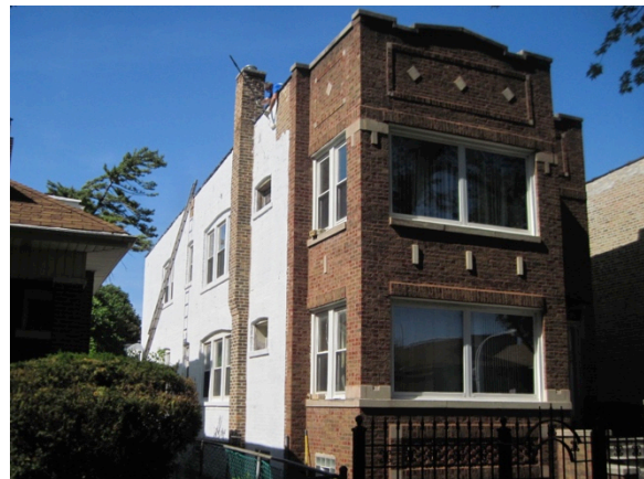
Figure 13. (L) Elastomeric paint application at larger multifamily building. Note that sills of windows are not painted; (R) Elastomeric paint application at two family building. (Credit: Scott Sanders, CEDA)
