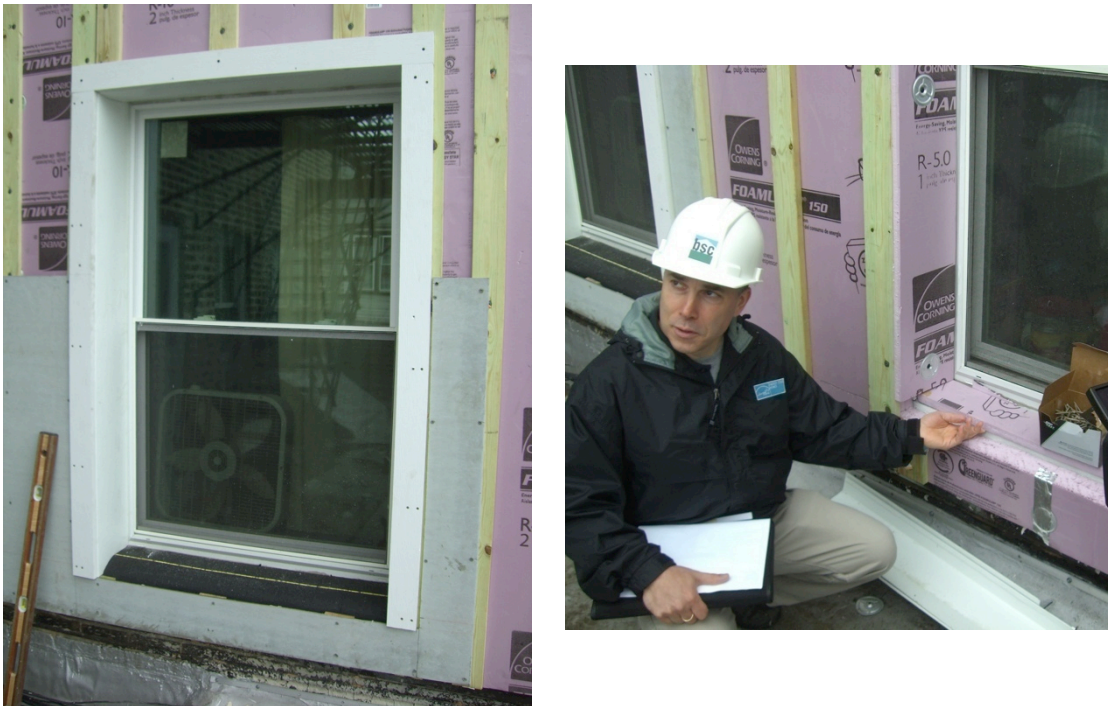
Figure 39. (L) Contractor mockup of window surround; (R) BSC personnel explaining placement of flashing membrane (Credit: John Yi, CEDA)
