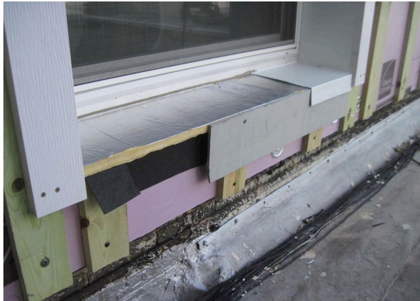
Figure 41. Second mockup of window surround showing the flashing membrane placed beneath the insulation return (Credit: Scott Sanders, CEDA)
