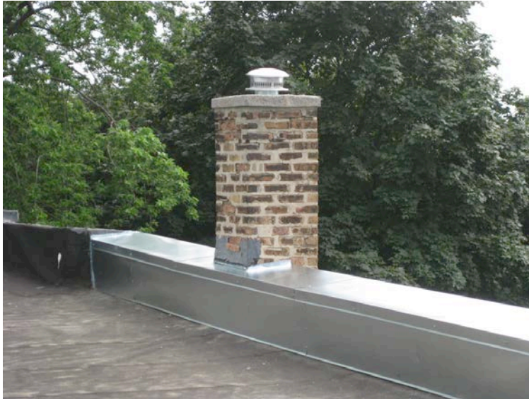
Figure 29. Finished parapet cover at two-family building
